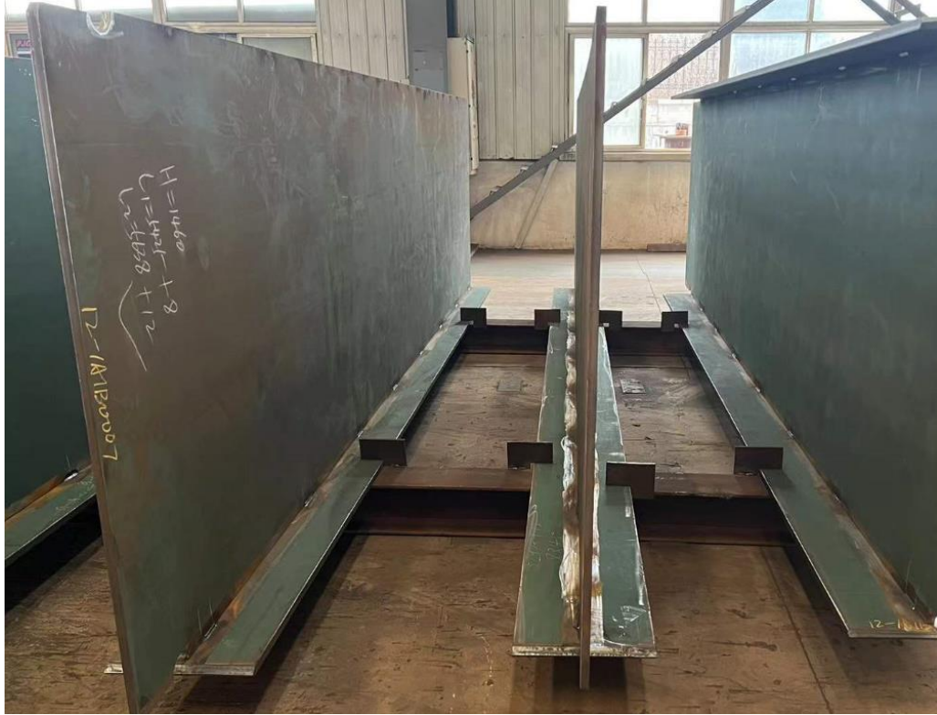
图7 PG梁防倾措施 c Fig.7 PG overturn-preventing c
